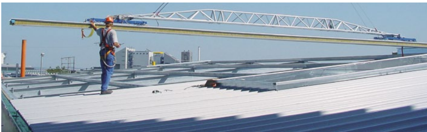
Example of roof assembly with traverse
