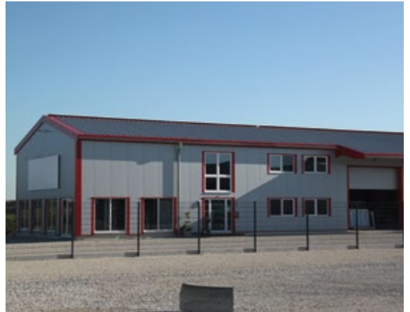
Production building with office
