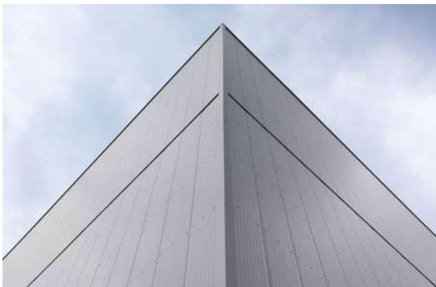
High-bay storage warehouse with panel laid vertically
